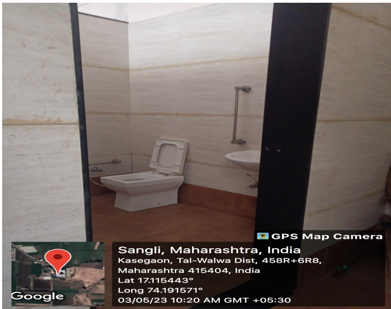
Ladies Toilet for Divyang
